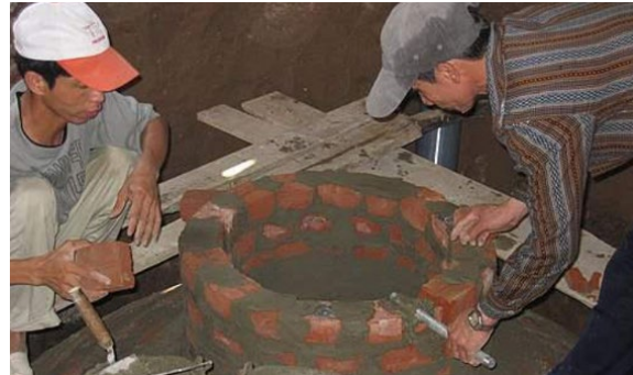
Figure 1B: Fixed-dome biogas plant. Source: Anaerobic Digestion Community, “Biogas Digester Facts.” (Anaerobic Digestion Community, 2018).
