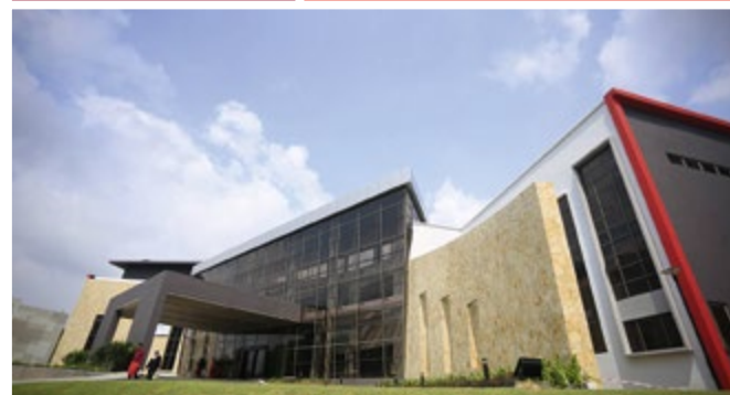
④ The new MIGHT building.
